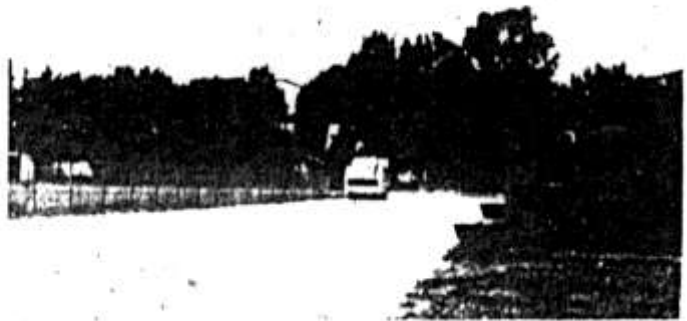
Rolling operations on freshly laid gravel were in progress Monday at Waggener's grid field, which was scheduled to be paved yesterday.
